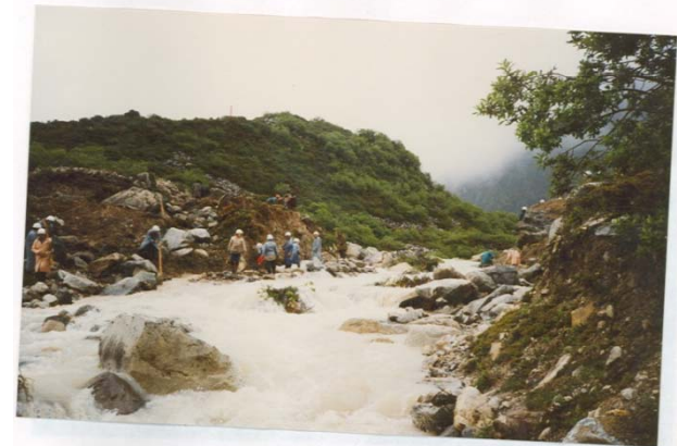
Fig. 4. 1 (b) WIDENING BETWEEN SUBSIDIARY LAKE I & II (WORK IN PROGRESS)
